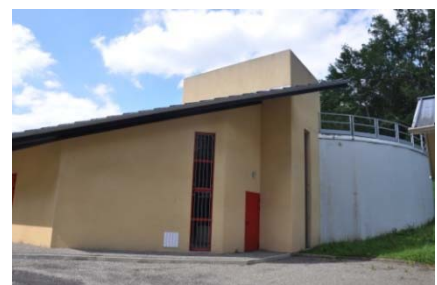
Photo 15 - Station de Bordes
