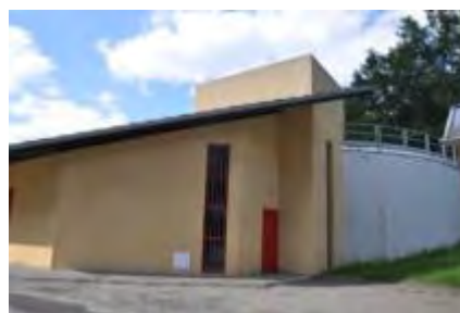
Photo 16 - Station de Bordes
