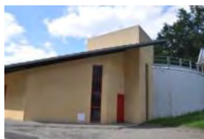
Photo 16 - Station de Bordes
