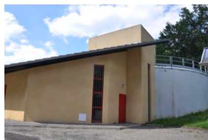
Photo 16 - Station de Bordes
